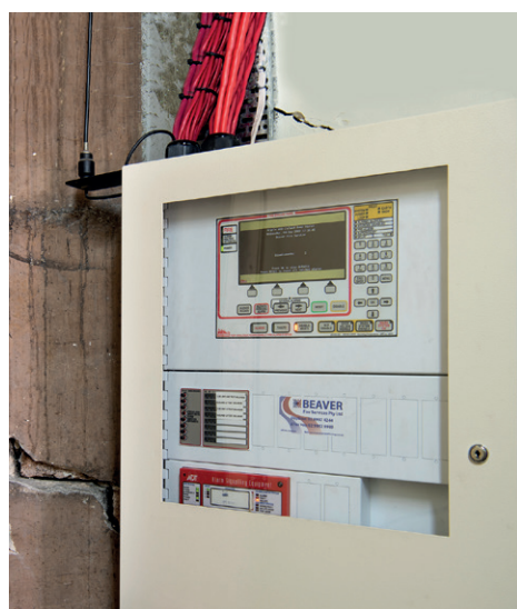
Top: The historic Argyle Stores building Above: Pertronic F220 fire alarm control panel at Argyle and Cleland Bond Stores
